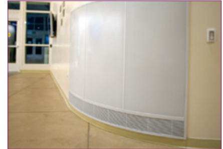
Figure 16: DF1W-HC, displacement diffusers with heat-cool changeover
