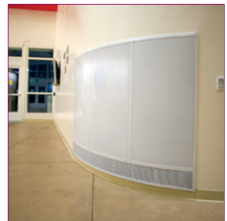
Figure 34: DF1W-HC installed in wall
