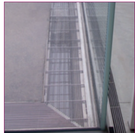
Figure 32: DFGL installed continuously along a perimeter
